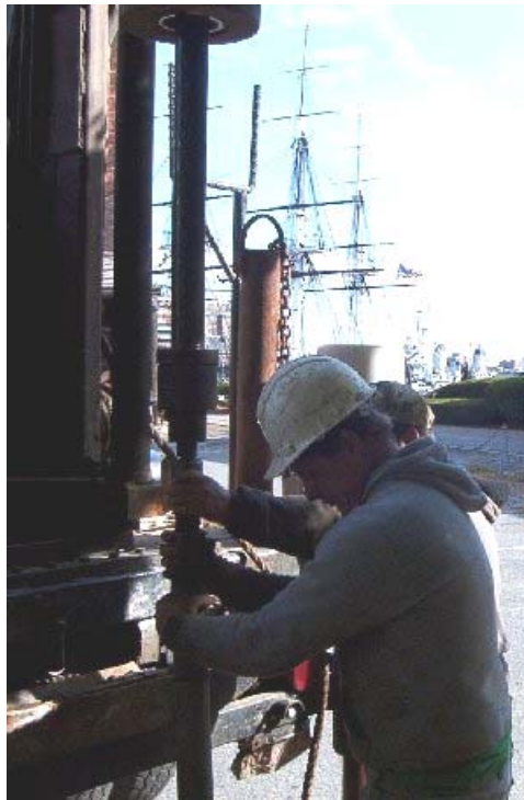
Photograph 2.2 – Standard Penetration Test
