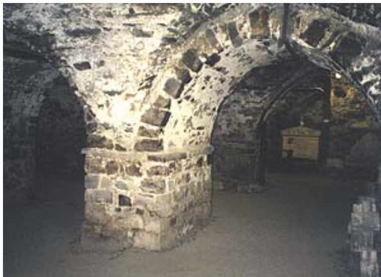
Photograph 1.1 - Foundations for a Medieval Era Cathedral
