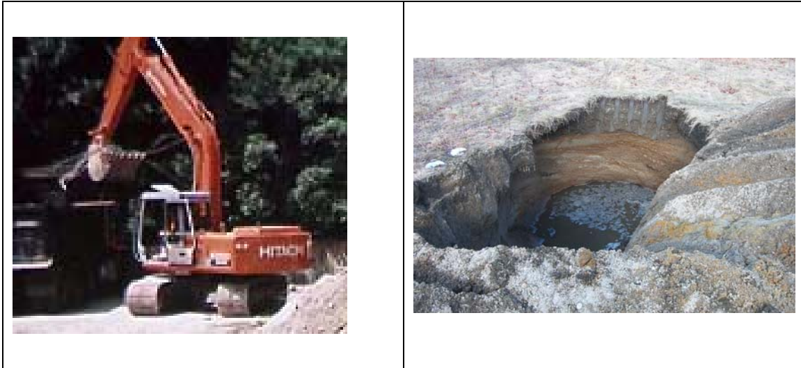
Photograph 2.1 – Test Pit Excavation
