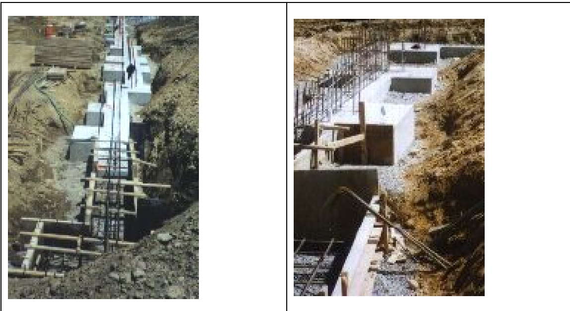
Photograph 4.1 – Shallow Spread Footings
